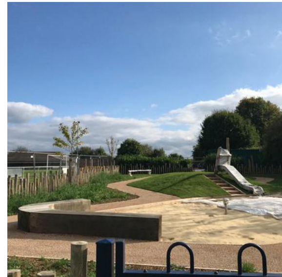
Colney Heath Play Area Prior to site completion
